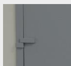
Anti-unhinging mechanism
